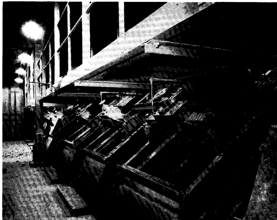
Granulation equipment is an important part of the Davison plant at Bartow, Fla. These screens in the Dorr granular process size the dried and pelletized products to exact specifications and return both oversize and undersize material
